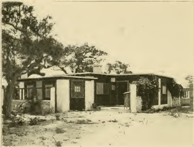
A UNIT OR PUEBLO HOUSE IN PROCESS OF CONSTRUCTION. CONCRETE ROOF AND CONCRETE FLOORS. THIS HOUSE CONSISTS OF THREE UNITS JOINED TOGETHER ON A TRIANGULAR LOT. VIEW FROM SOUTHWEST.
